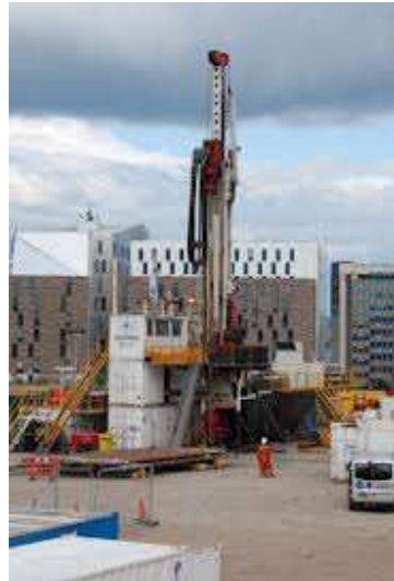
Drilling rig, Science Central site, Newcastle
